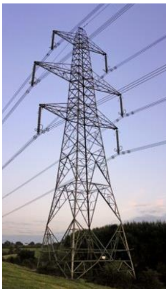
Image 5.10 Typical suspension steel lattice pylon 1
