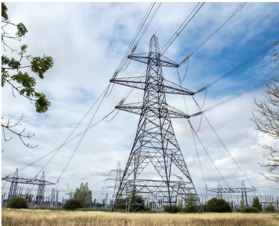
Image 5.13 Typical terminal lattice pylon 3
